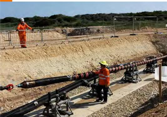
Figure 27. Horizontal Directional Drilling (HDD) Operations (Courtesy, Dudgeon Offshore Wind Farm).
