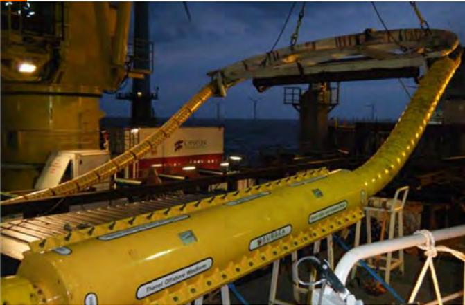
Figure 31. Lifting Cable Repair Joint with External Cable Protection (Courtesy, NKT Cables).
