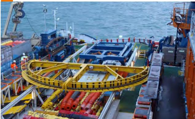
**Figure 41. Second-End Array Cable Installation, Quadrant Being Deployed, ROV in the Water** (Courtesy, Deutsche Buch Windfarm).
