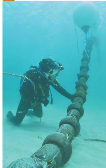
Figure 71. Urduct® Cable Protection (Courtesy, Trelleborg).
