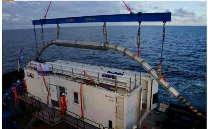
Figure 32. Deploying Cable Repair Joint (Courtesy, NKT Cables).
