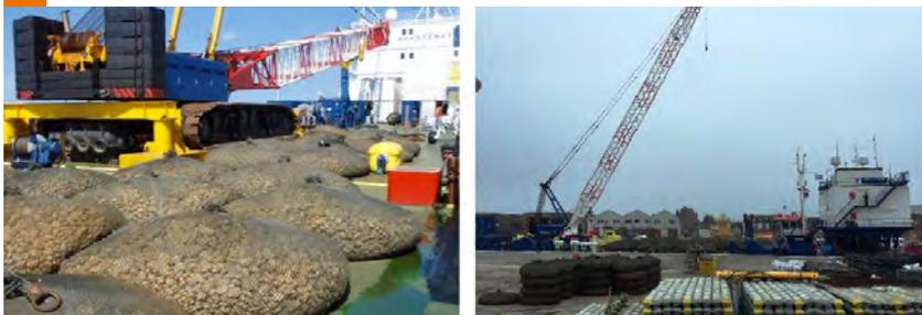
**Figure 75. Filter Bag Deployed** (Courtesy, Rockbags; rockbags.co.uk).
